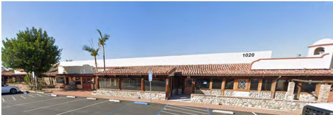
Above – photo of existing buildings at Old California Restaurant Row
